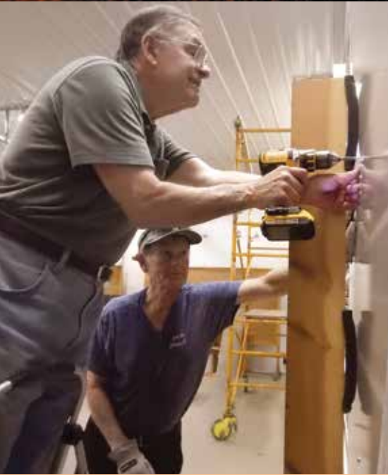
Volunteers Al Giannantonio and John Walker finish installing the train wall.
